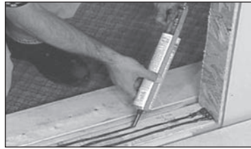
(Fig. 1-2) Caulking the sub-floor.
