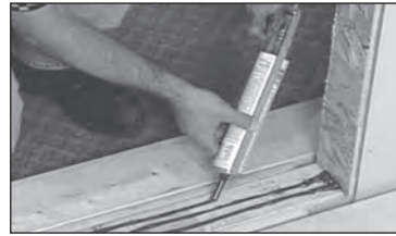
(Fig. 1-2) Caulking the sub-floor.
